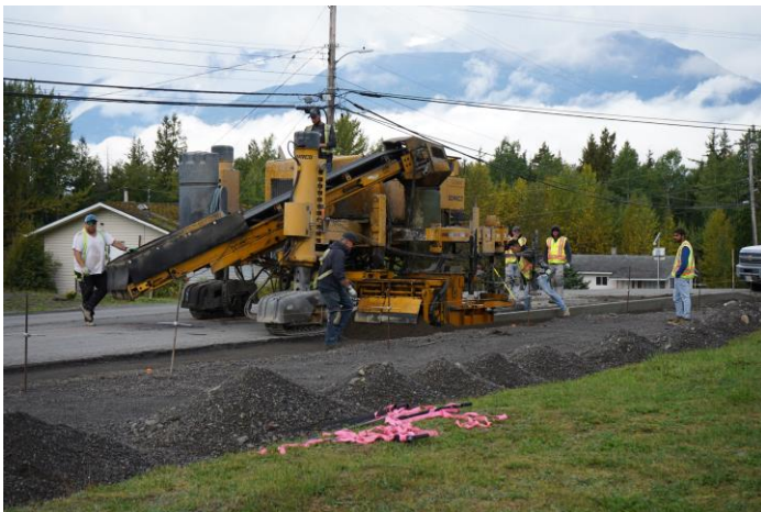
Skateen Sidewalk Curb being formed.
