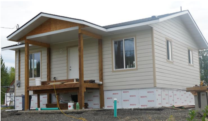
One of the six buildings that will comprise the Tiny Town Project.
