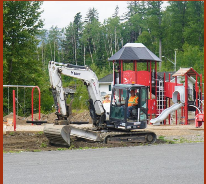
Landscaping begins at the water park near the Rec Centre.
